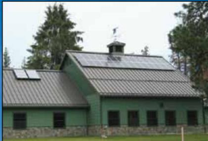
Both a solar hot water heater (panels on left side of roof) and 4.9 kW solar PV array (panels on right) provide clean and green power to the wildlife refuge facility.
